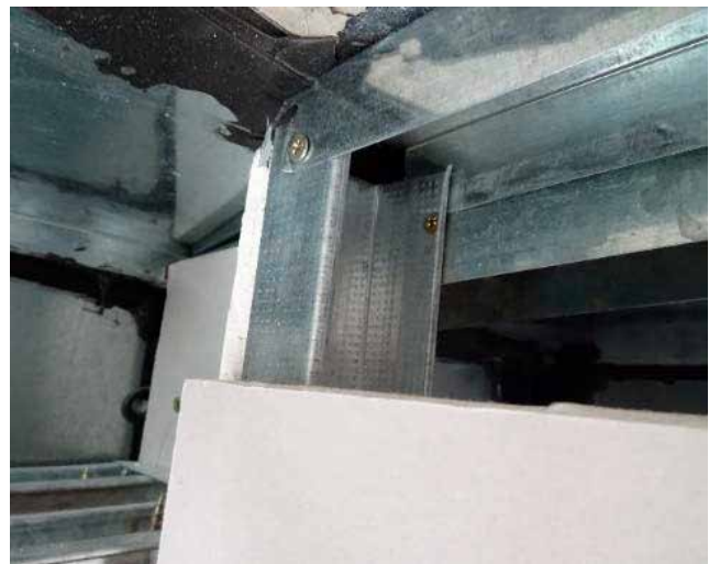
■ STEEL STUD FIXED INTO HEAD TRACK
