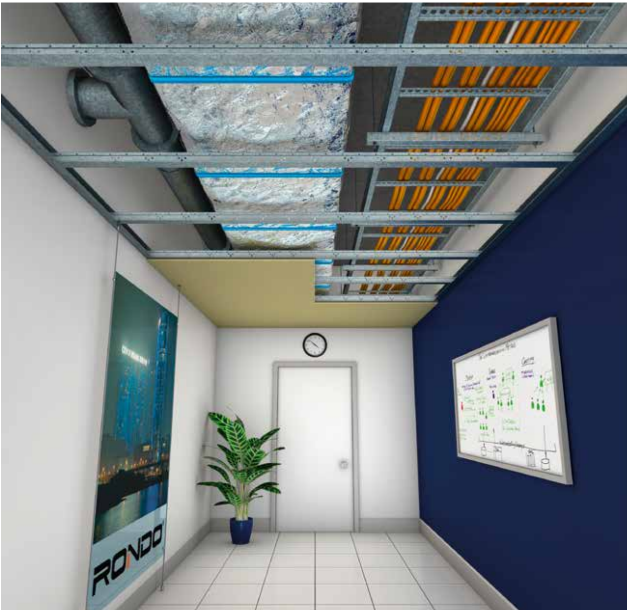
■ TYPICAL APPLICATION RONDRO XPRESS® DRYWALL CORRIDOR
